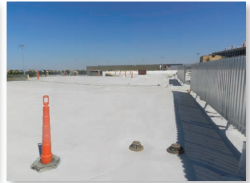
Step 3: Spray apply Coating
